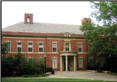
Hudson Hall 1948 87,022 sf Office of Horace Trumbauer Pratt School of Engineering 100,551 sf
