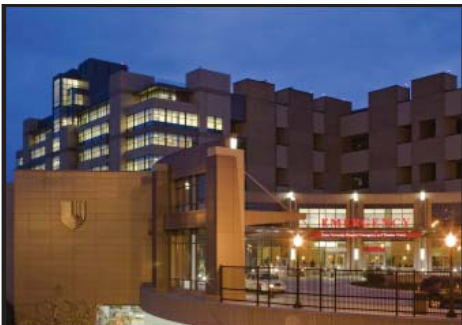
Emergency Department Expansion 2007 Perkins Eastman Hospital 56,770 sf
