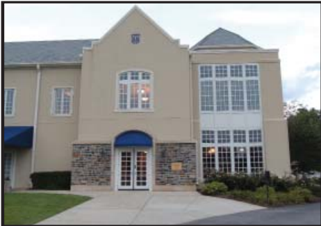
The Karcher-Ingram Golf Center 2005 Rabun Architects Golf Team Facility 5,500 sf
