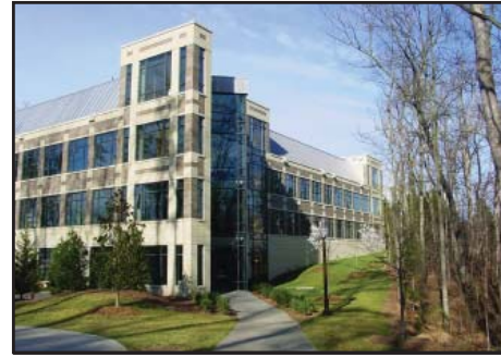
Rubenstein Hall 2004 Architectural Resources Cambridge Inc Sanford School of Public Policy 66,446 sf LEED Certified
