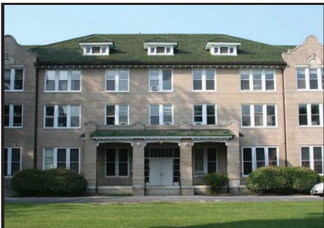
Southgate Residence Hall 1921 C.C. Hook Student Residence (158 Beds) 47,712 sf
