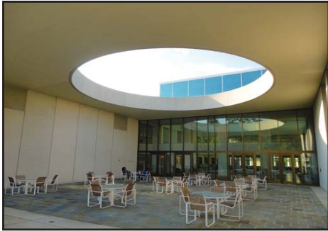
Thomas Keller Center Entry and Courtyard
