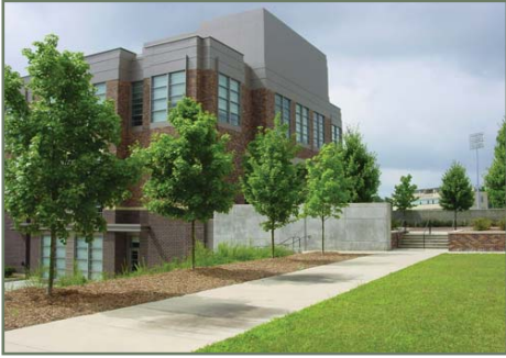
Yoh Football Entry Plaza and Courtyard
