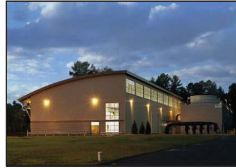
Chilled Water Plant #2 2005 Woolpert Chilled Water Production 63,717 sf
