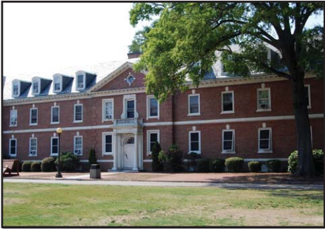
Giles Residence Hall 1928 Office of Horace Trumbauer Student Residence (127 Beds) 45,557 sf
