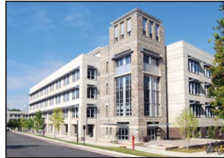
Medical Science Research Building II 2006 Hillier Architecture Research and Offices 168,701 sf LEED Silver
