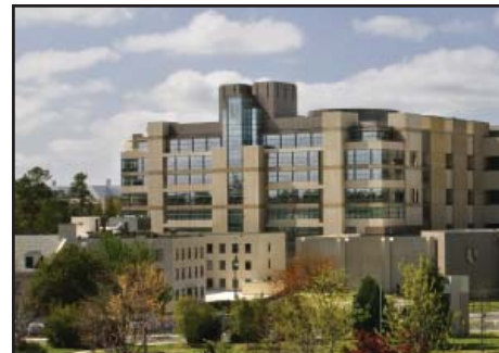
Hospital Addition for Surgery (HAFS) 2008 Perkins Eastman/Duda Paine Hospital 133,000 sf
