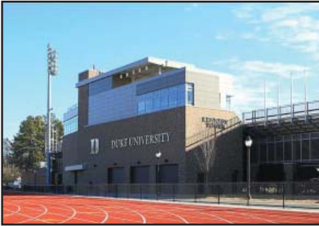
Williams Track & Field and Kennedy Tower 2015 CHA Sports Track & Field Stadium/Media Tower 12,000 sf
