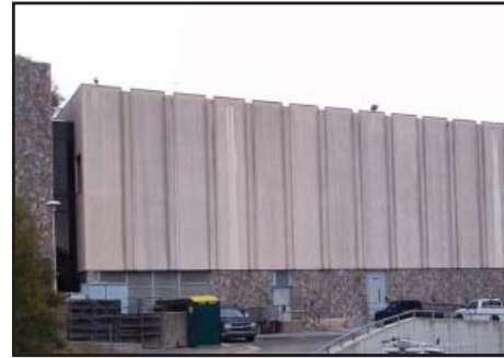
Telcom Building 1973 J.N. Pease Associates Office of Information Technology 26,680 sf
