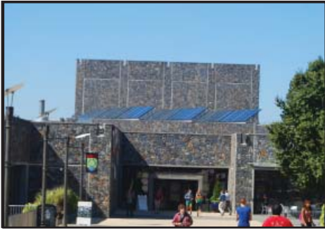
Bryan Center 1982 Hayes-Howell Associates/ Caudill, Rowlett & Scott Student Support 217,887 sf
