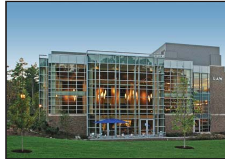
Star Commons at Duke Law 2008 Shepley Bulfinch Law School 6,500 sf LEED Certified
