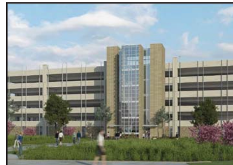
Science Drive/Cameron Blvd. Parking Garage 2017 Walker Parking/Ratio Architects Parking Deck (2,320 spaces) 824,800 sf
