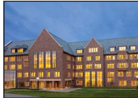
Keohane Quad 4E 2011 William Rawn Associates Student Residence (149 Beds) 71,000 sf LEED Silver
