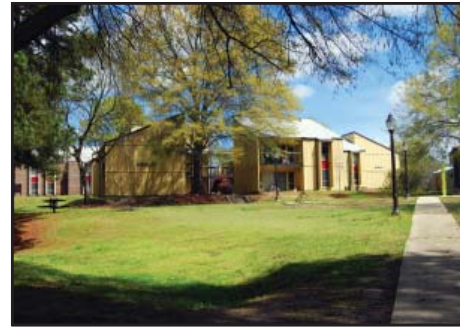
Central Campus Apartments Renovations 2010 J Davis Architects Student Residence (1055 Beds) 415,155 sf
