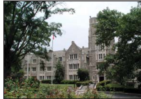
Allen Building 1954 Office of Horace Trumbauer Administration Office and Classroom Space 73,575 sf
