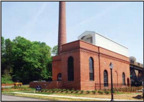
East Campus Steam Plant 2010 Smith Group JJR Steam Production 13,598 sf LEED Gold
