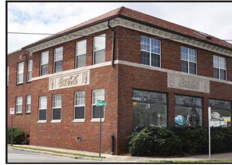
Bevan Building 2004 Offices 18,515 sf Architect Unknown 1930
