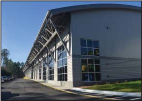
Chilled Water Plant #2 Addition 2011 FLAD Architects Chilled Water Production 31,000 sf LEED Gold
