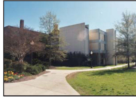
Hudson Hall Annex 1973 Caudill, Rowlett & Scott Pratt School of Engineering 30,000 sf
