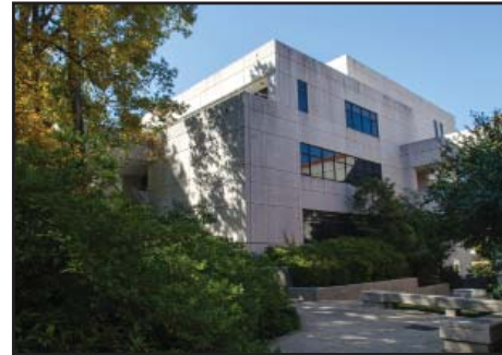
Nello L. Teer Building 1984 Nicholson Architects Pratt School of Engineering 43,362 sf
