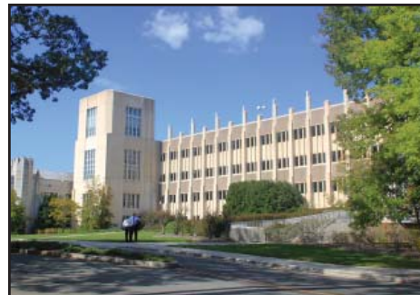
Parking Garage for Duke Clinic 1995 Cooper Robertson and Partners Parking Deck (1,794 spaces) 594,916 sf
