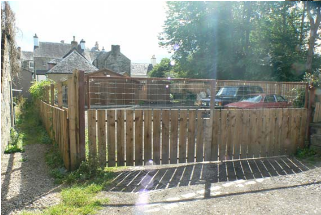
Boundary fencing to the rear of Atholl Street's commercial properties
