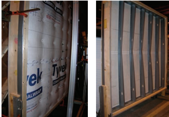
Figure 6. Phase II: Structural High Pressure Performance Testing
