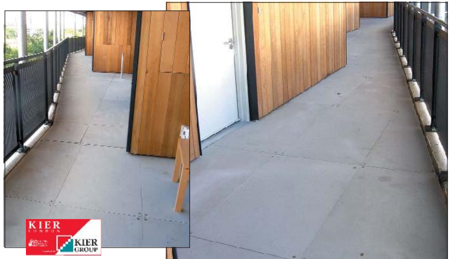
Dura Slab was used on several floors of this residential development
