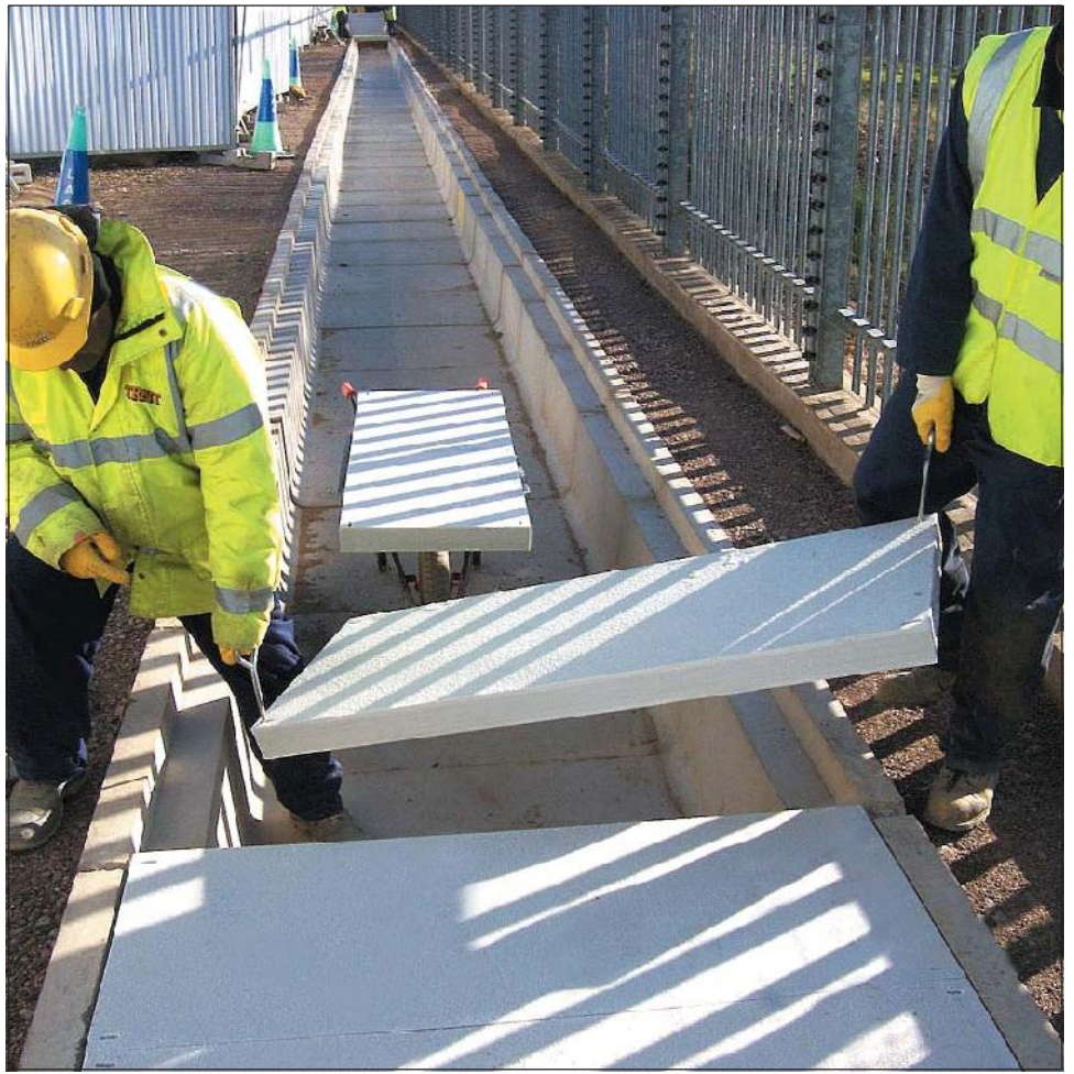
Installation process made easy through lightweight panels and lifting keys
