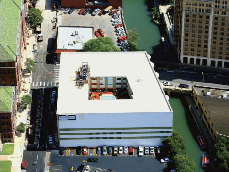
Riverwalk Plaza Hotel San Antonio, TX
