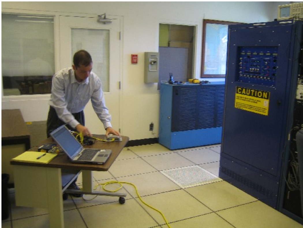
Figure 5-5: Bench testing the AP in the King Site radar control room.
