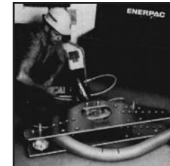
Pipe is ejected hydraulically.
