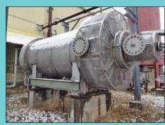
Process Combustion Corp 400MM BTU / Hour Industrial Air Heater
