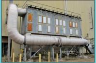
\*\*Dust Collector, 53 Ton Storage Silo, 5.3M BTU/Hr. Air Heater, Blowers
