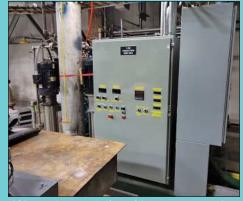
Skid Mount Pump Station with 25 HP Pump and PLC Controls
