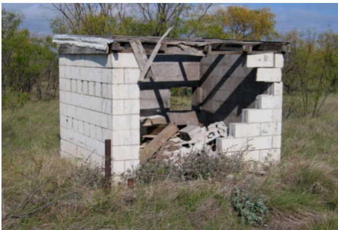
The remains of skeet field 1 low house, and the most intact portion of property. The target opening is clearly visible on the far wall. The houses were well built of concrete block construction. Manual traps were in place during the early years, later replaced with “modern” electric models.
