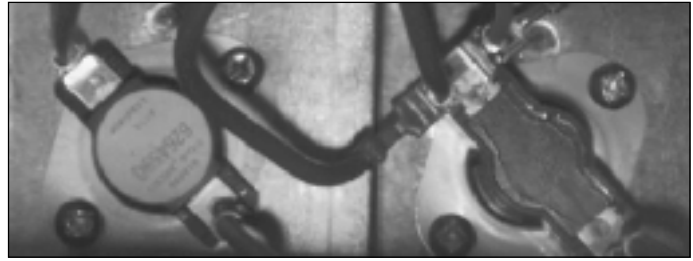
Figure 7. Limits in furnace
