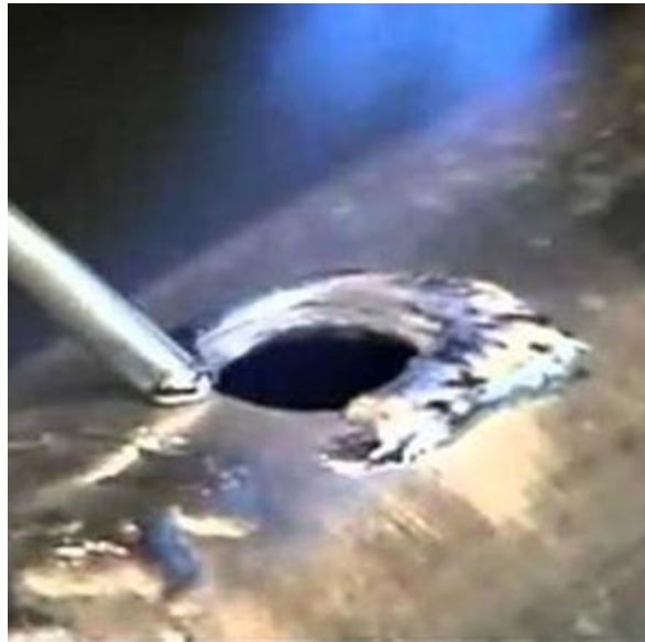
Repair soldering of a hole in an aluminium pipe
