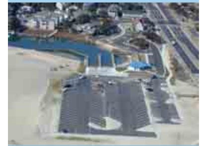
The Lynnhaven Boat Ramp and Beach Use Facility
