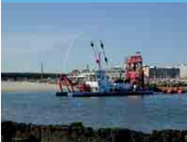
Rudee Inlet II dredging in the Sand Trap
