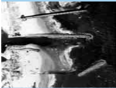
Rudee Inlet immediately after infrastructure improvements, March 1968
