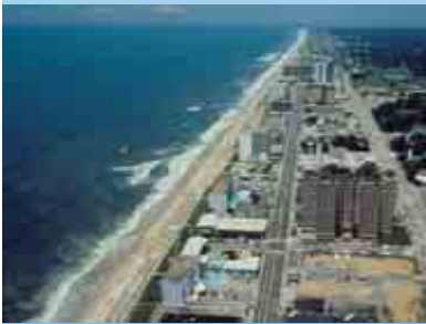
Before beach replenishment in 1998
