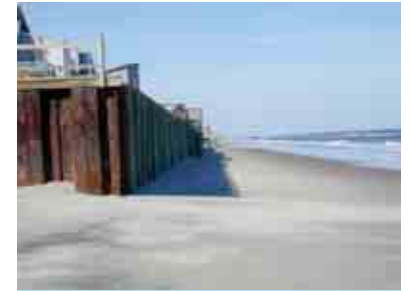
Bulkhead at Sandbridge Beach
