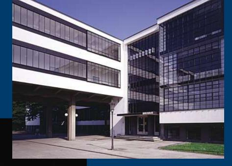
• projected steel skeleton, which pulled the function of support to the inside
