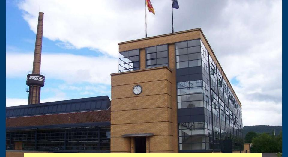
**Curtain Wall**: Nonbearing wall of glass, metal, or masonry attached to a building's exterior structural frame.
