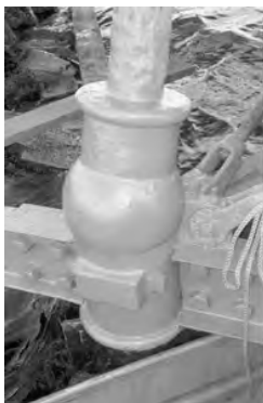
Cast iron coupling at Thomas Point Lighthouse
