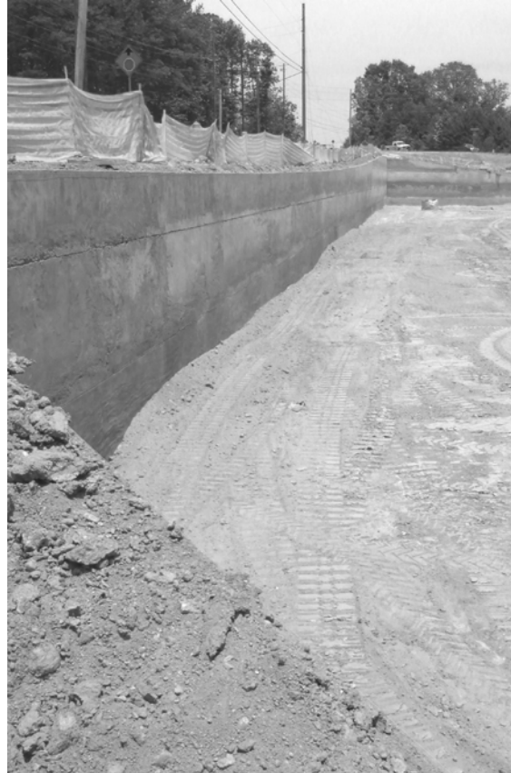
A view of a finished ECP Soil Nail retaining wall.
