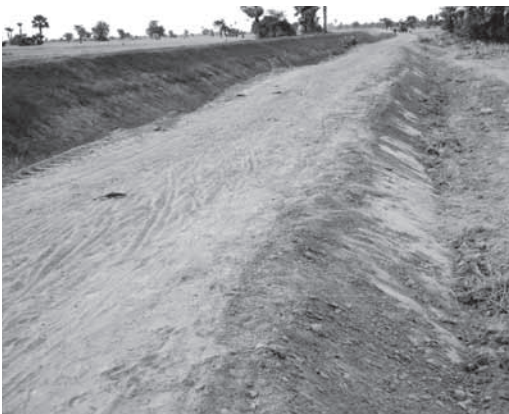
The ox cart path situation before (L) and after (R) one season of operation showing severe rainy season damage.
