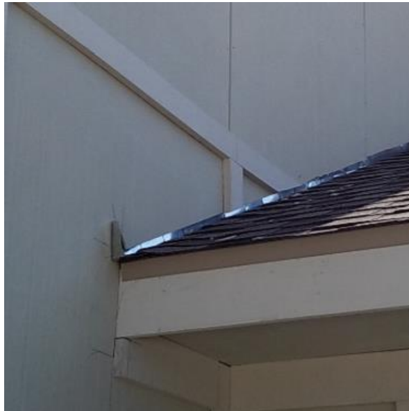
Flashing installed properly between roof and exterior wall.
