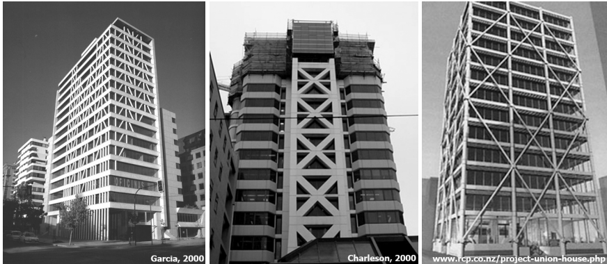
Figure 3: Example of cooperation between architecture and earthquake engineering: Manantiales building, Chile (left), Wool House in Wellington (middle) and Union House in Auckland with added bracings (right).
