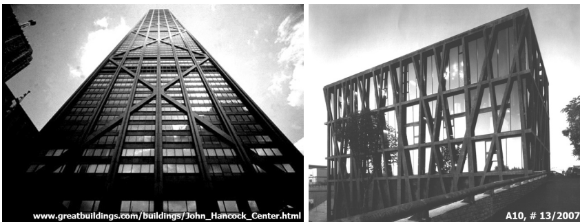
Figure 4: Example of identification of architecture with seismic design: tectonic (trapezoidal) shape of Hancock Building in Chicago with visible bracings over the facade (left) and Dance centre Aix-en-Provence (right).
