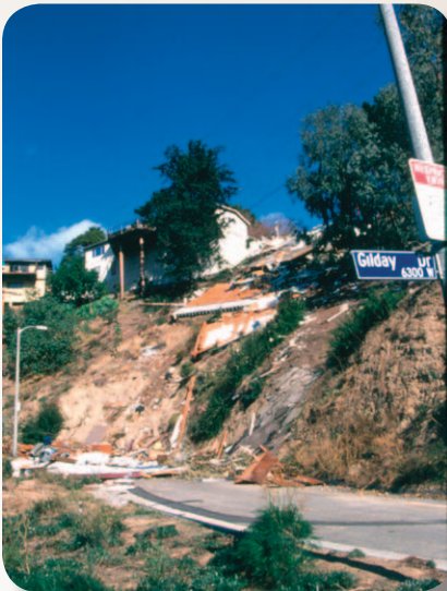
Figure 13. Landslide generated during the 1994 Northridge, California, earthquake (image courtesy of FEMA).
