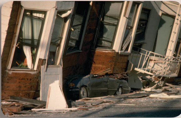
Figure 14. Building in San Francisco's Marina section that foundered as shaking from the 1989 Loma Prieta earthquake caused liquefaction (image by U.S. Geological Survey).
