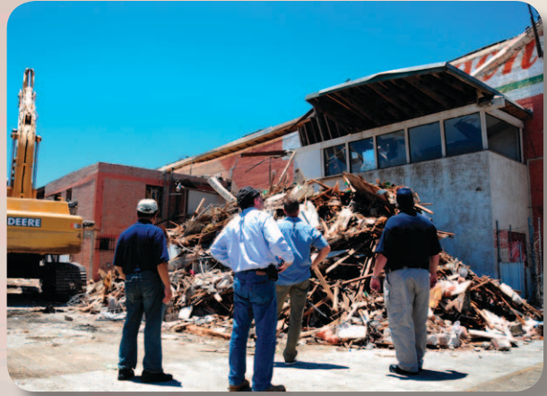
Figure 11. Building in Calexico, Mexico, damaged during 4 April 2010 El Mayor earthquake (image by Adam Dubrowa, Federal Emergency Management Agency).
