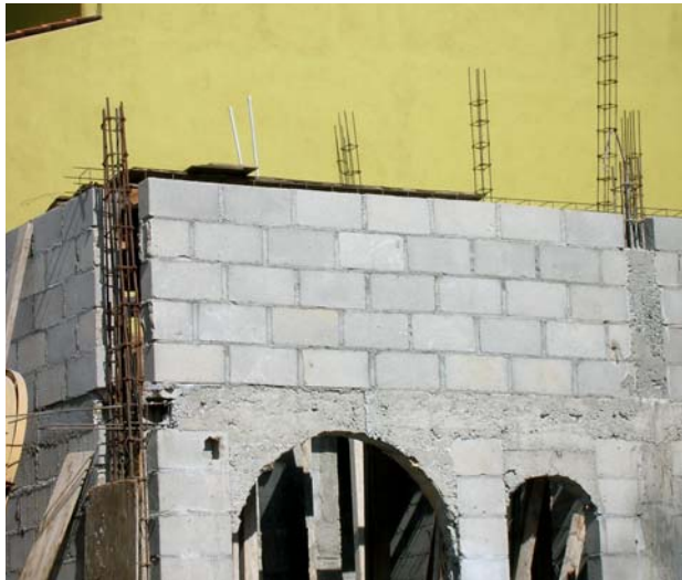
Figure 5. Examples of RC frame construction in Cambodia (top) and confined masonry construction in Mexico (bottom) 1
