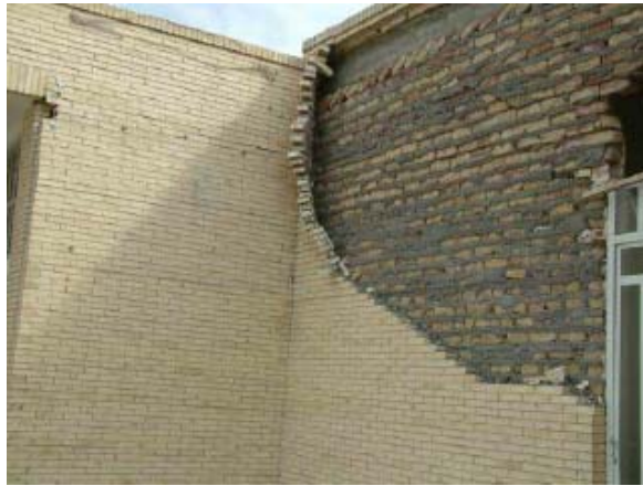
Figure 22. Damage to the confined masonry construction in Iran due to the 1990 Manjil earthquake 9 (top) and the 2003 Bam earthquake 10 (bottom) (note that the absence of a tie-column at the door jamb on the latter photo)
