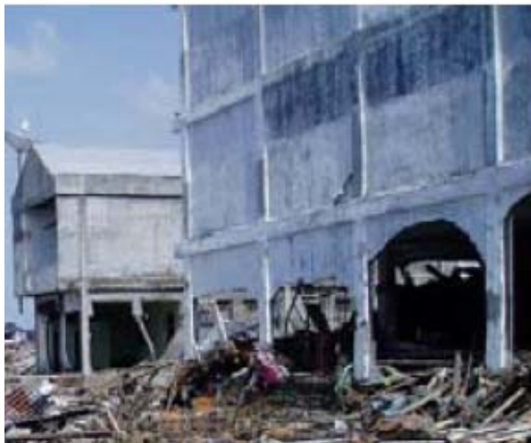
Figure 23. Confined masonry buildings in Banda Aceh, Indonesia, after the 2004 Great Sumatra earthquake and Indian Ocean tsunami 11 : good performance of confined masonry in the midst of devastation (top), and tsunami-induced out-of-plane failure of masonry walls at the ground floor level (bottom).
