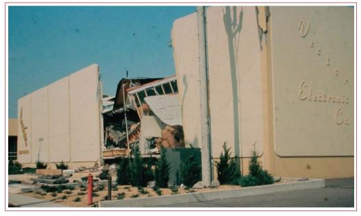
Figure 16 Collapse of a tilt-up building in the 1971 San Fernando earthquake (photo by P. Yanev).
