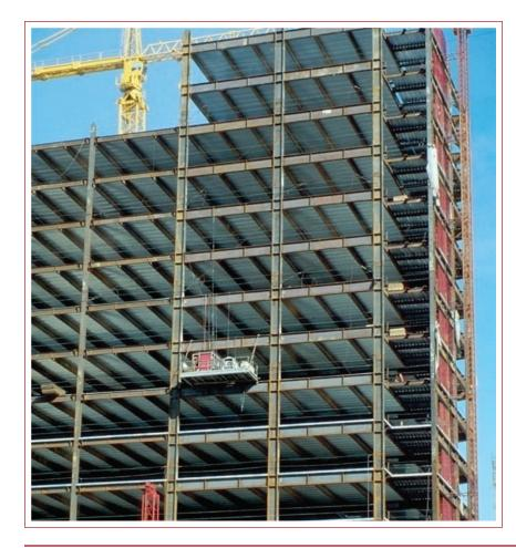
Figure 25 A tall steel moment-frame structure under construction.
