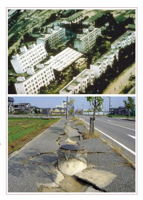
shows liquefactioninduced settlement of apartment buildings in the 1964 earthquake in Nigata, Japan (photo courtesy of the University of Washington). The bottom photo shows one of many manholes that floated to the surface as a result of soil liquefaction caused by the 2004 Chuetsu earthquake near Nigata, Japan (photo courtesy of Wikimedia Commons).
