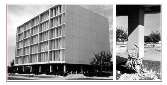
This six-story structure had several types of irregularity including end shear walls that stopped below the second floor and a first story with less strength and stiffness than the stories above. As a result, earthquake energy dissipation and damage were concentrated in the first story columns, a condition that could not be repaired and required demolition of the building after the earthquake. In a more severe earthquake, this type of damage could have caused the building to collapse.
