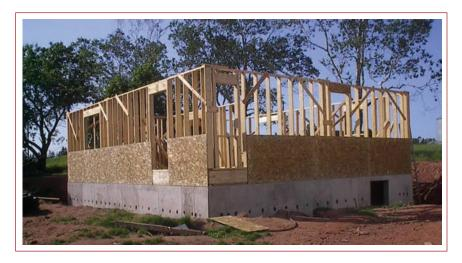
Figure 21 Wood studs and structural panel sheathing of typical wood frame bearing wall construction.
