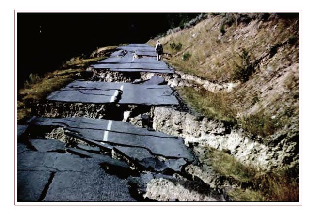
Figure 7 Lateral spreading damage to highway pavement near Yellowstone Park resulting from the 1959 Hegben Lake earthquake (photo courtesy of the USGS).
