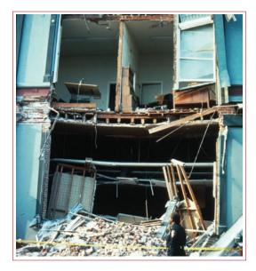
Figure 20 Failure of an unreinforced masonry wall in a building in Santa Cruz, California, in the 1989 Loma Prieta earthquake.
