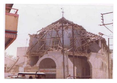
Plate 1: Out-of-plane flexure failure
