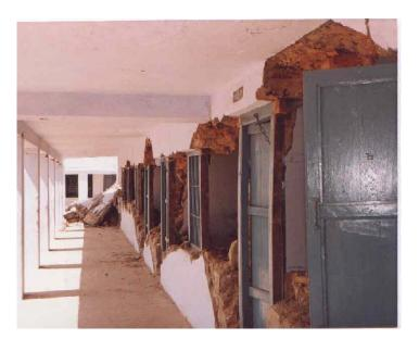
Plate 3: Failure of masonry piers between openings
