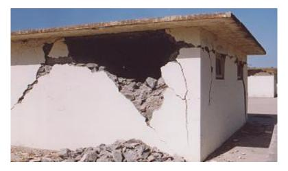
Plate 6: Separation of roof from walls
