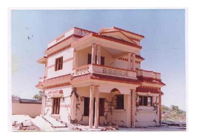
Plate 10.6: In-plane shear failure
