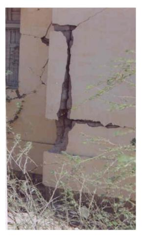
Plate 2: Separation of wall at junctions
