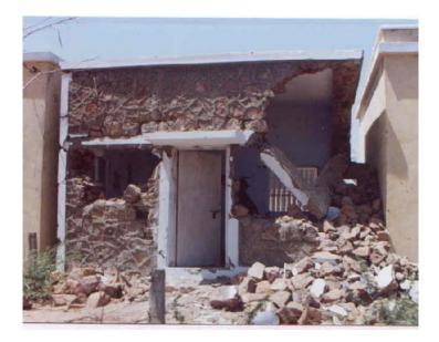
Plate 4: Local failures
