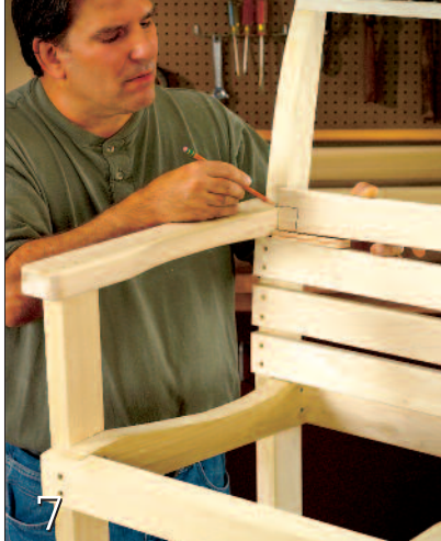
7 Mark the position of the armrests on the fourth back slat. Cut notches in the back slat to fit around the armrests.
