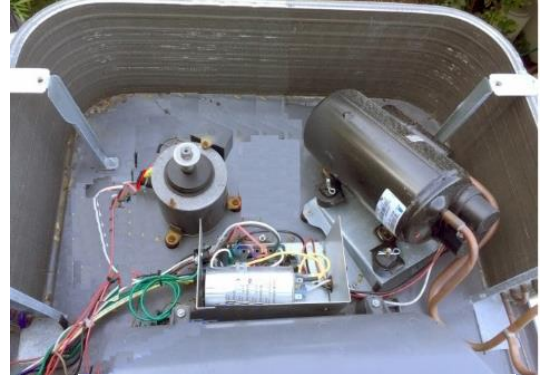
Figure 11: Early Mach 8 (style 1) with capacitors inside electric box
