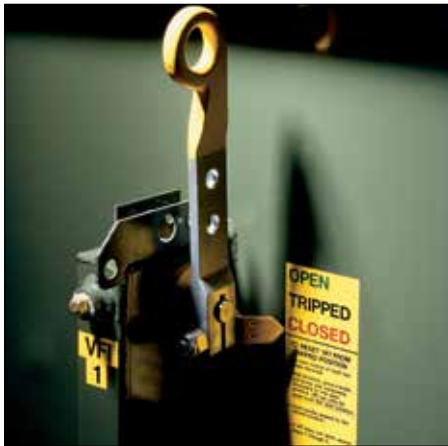
Figure 13. VFI—operating handle.
