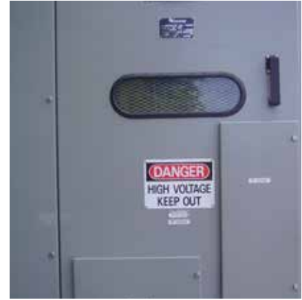
Figure 18. LIS—switch position viewing window.
