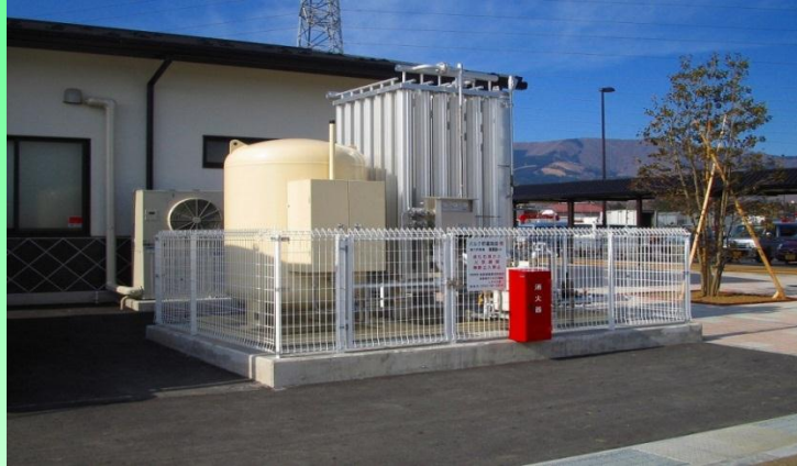
Installation for GHP & Restaurant Kitchen
