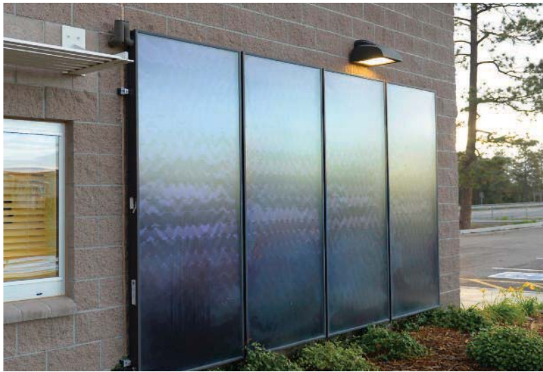
The solar collectors are mounted vertically and integrated into the building's architecture. This orientation provides more space heat in winter when the heat is needed most and minimizes the possibility of overheating in the summer.
