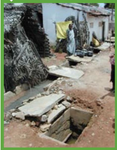
Water well (right) adjacent to an open sewer.
