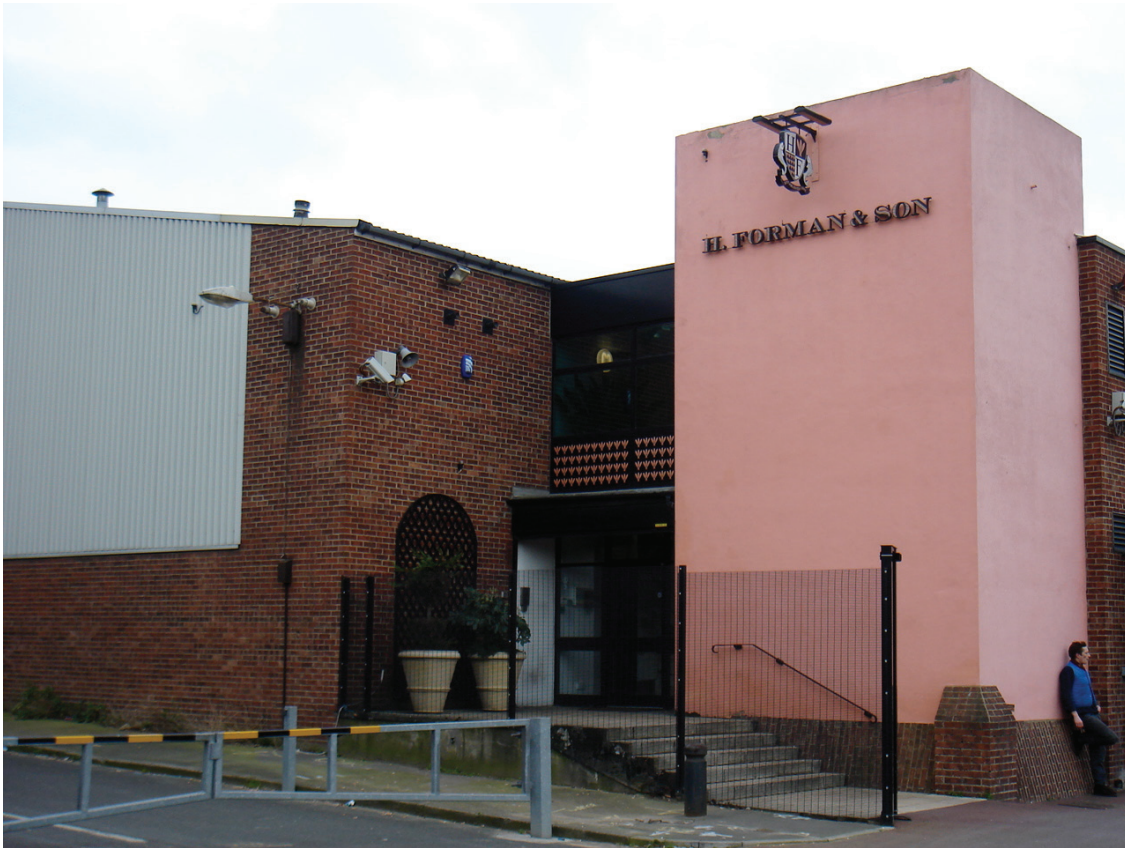
Figure 11 – Forman's smoked salmon factory in 2007, now demolished
