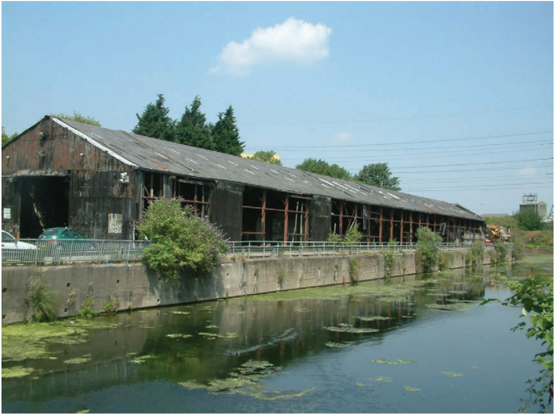
Figure 15 – An abandoned factory which had to be cleared for the new Olympic Park
