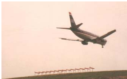
Localizer antenna array for instrument landing system.
