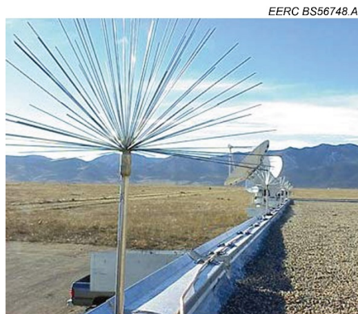
Figure 4. Example of CTS air terminal (source: Lightning Eliminators).
