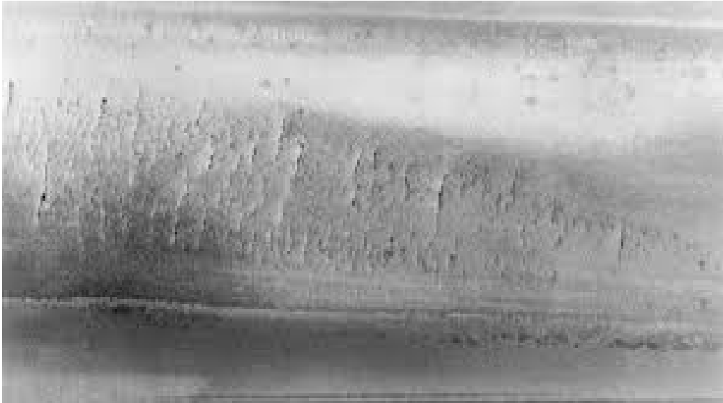
Fig.2 Stress corrosion cracking in pipe[3]
