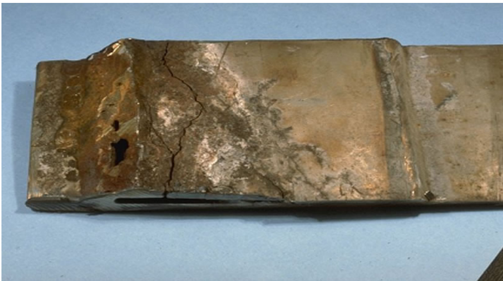
Fig.3 Stress corrosion cracking in material
