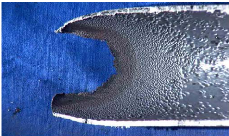
Fig.1 Flow Accelerated Corrosion
