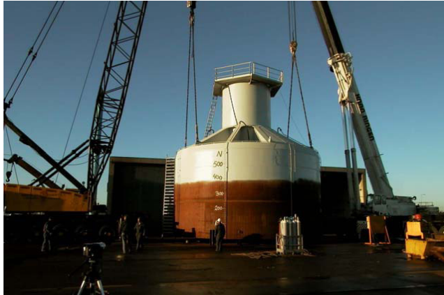
Figure 4. Bucket foundation for Vestas 3MW wind turbine in Frederikshavn
