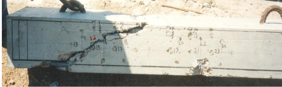
Figure 2 a: Shear Cracks on beam (A 0 ); Sudden Shear Failure
