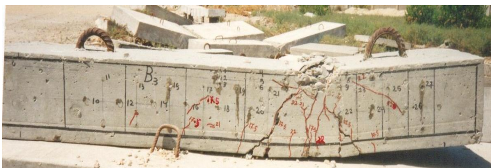
Figure 3 d: Shear Cracks on beam (B 3 ); Flexure Failure
