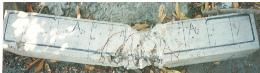
Figure 2 c: Shear Cracks on beam (A 2 ); Flexure Failure
