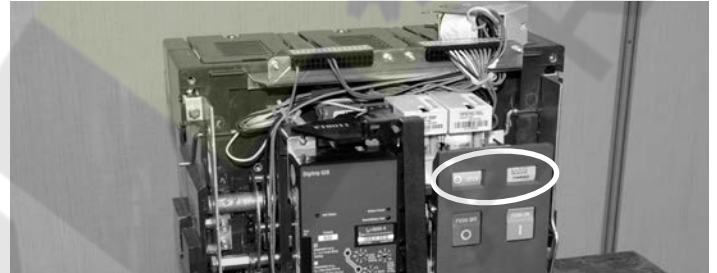
Figure 110. Charged and opened
