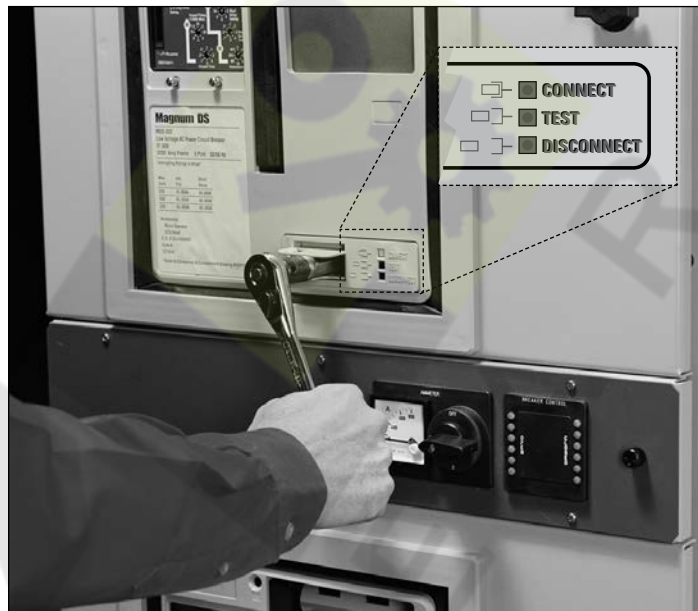
Figure 16. Levering position indication
