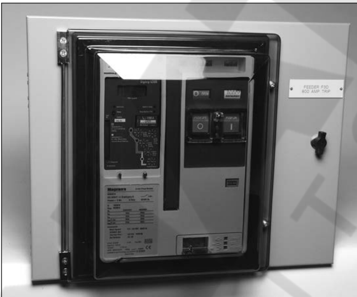
Figure 59. IP55 waterproof cover
