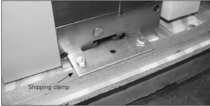
Figure 6. Shipping clamps for drawout circuit breaker
