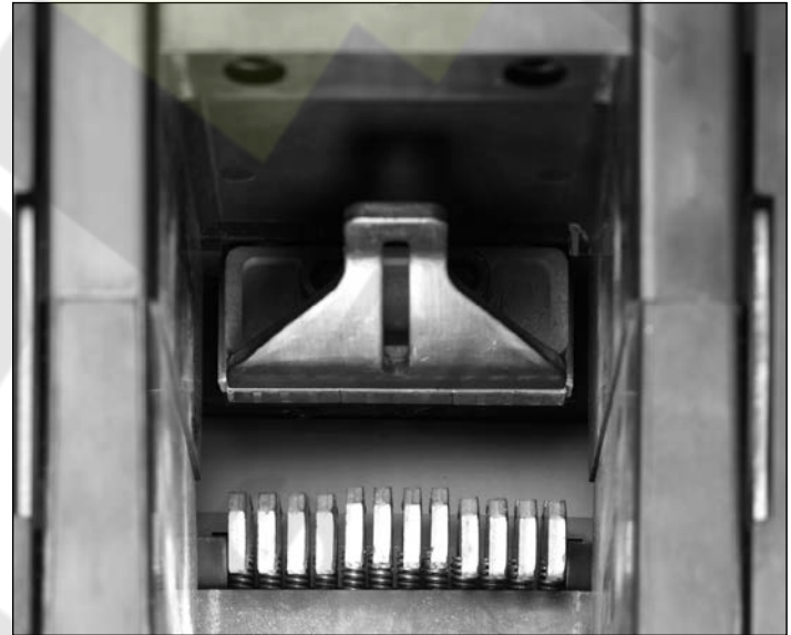
Figure 98. Primary contacts with circuit breaker open (not used for contact wear inspection)
