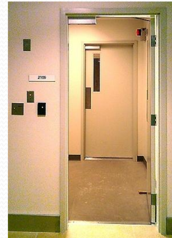
Mantrap Shield in airlock converted from a small room
