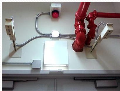
Model DS200 installation in a high ceiling location using wall brackets.
