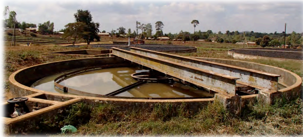
Figure 5: One out of two sedimentation tanks at the municipal WWTP.
