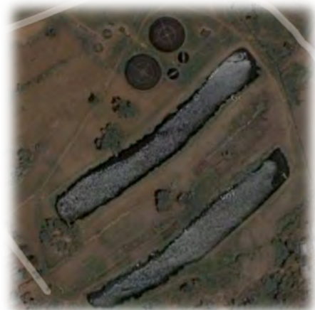
Figure 3: View of Zomba WWTP. The two maturation ponds shown in the picture are about 150 m long (Google Map Maker, 2012).
