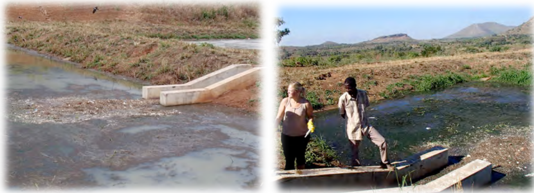
Figure 12: Fifth pond that should normally work as the first of two maturation ponds at the Chancellor College. By time of sampling the function of the pond was more similar to that of a facultative pond.
