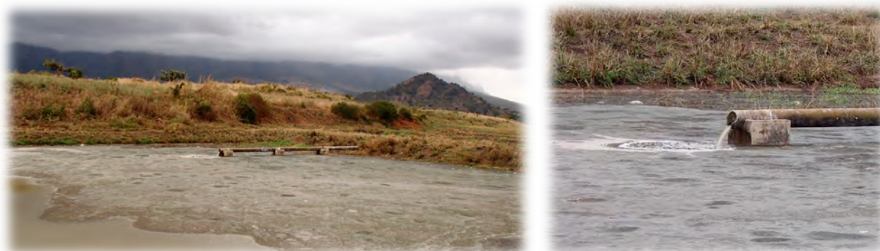
Figure 11: Fourth pond normally working as a second facultative pond at the Chancellor College. By time of sampling, serving as anaerobic pond
