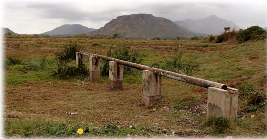
Figure 9: The inlet pipe to the first anaerobic pond at the Chancellor College WWTP. By time of sampling, this pond was not working and no water was stored there.
