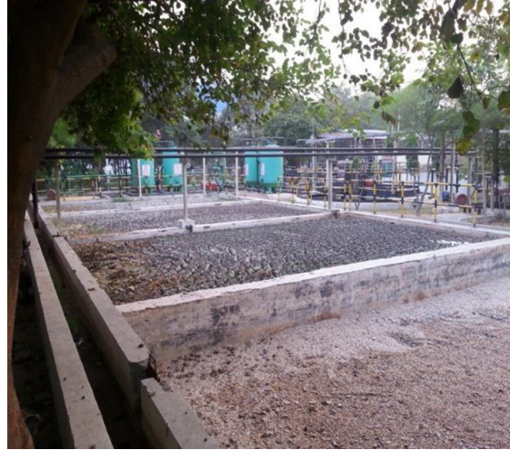
Better filtration of sludge after intervention
