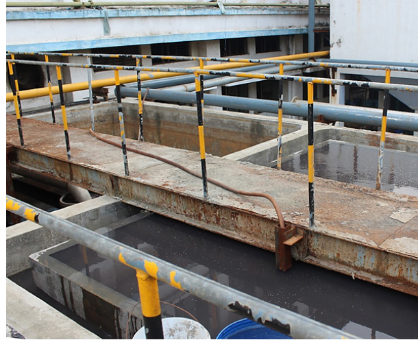
Large-scale textile company removed the problems in the settling of solids in the ETPs clarification tanks due to insufficient capacity of clarifier tanks by increasing the increase the capacities of the Primary and Secondary Clarifiers.
