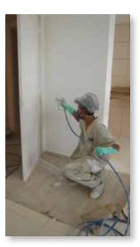
With a 2.4 hp brushless DC motor and the ability to spray up to 4.5 liters per minute, the Ultra Max II 1095 is the industry standard for the large residential and commercial contractor who sprays a wide variety of coatings.
