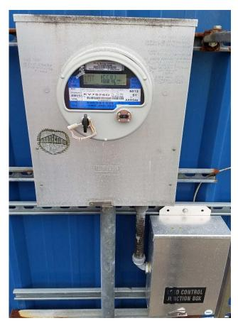
Figure 1. FSEC Facility Electric Meter and Junction Box Access to Switch Mechanism
