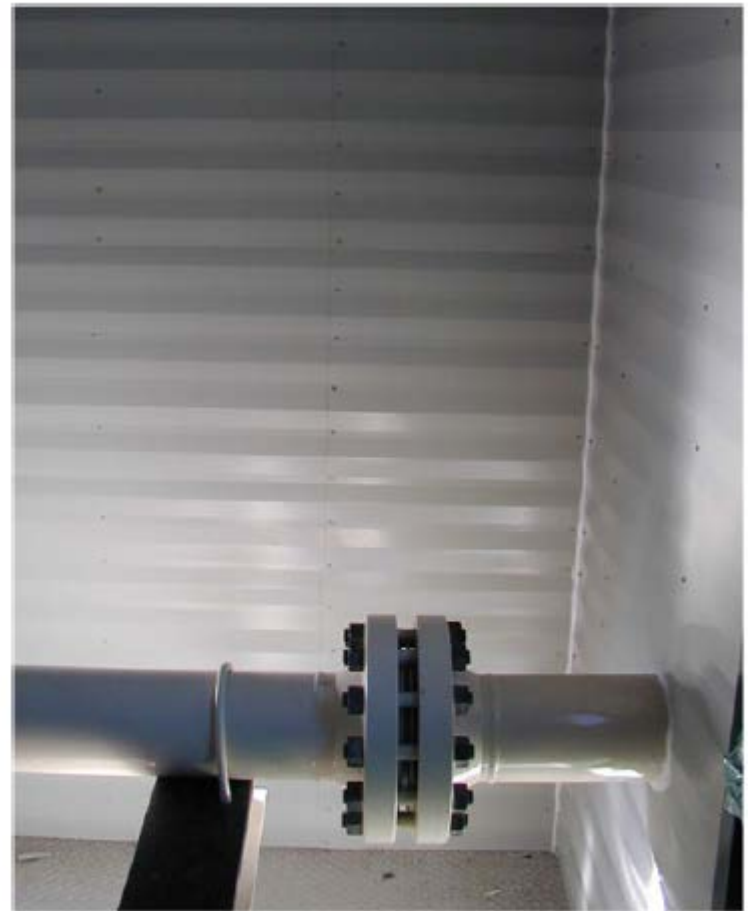
Fig. 13. Pipe wall penetration sealed.
