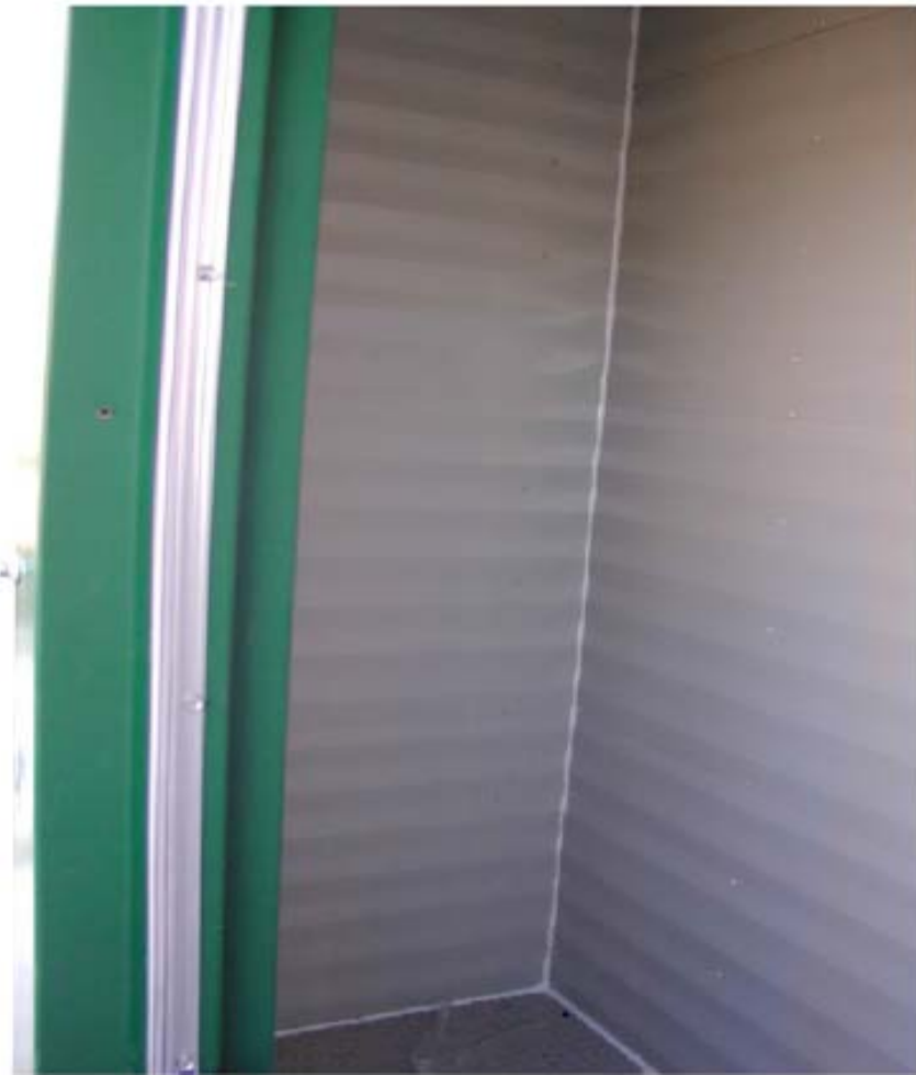
Fig. 12. Walls showing joints with caulking.
