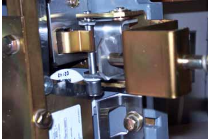
Figure 9 – Mechanical Latch Mechanism Adjustment (as viewed from the front with contactor resting on the left side)
