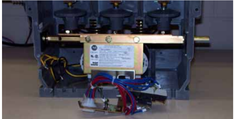
Figure 3 – Disconnecting Coil Leads from Auxiliary Contact Assembly
