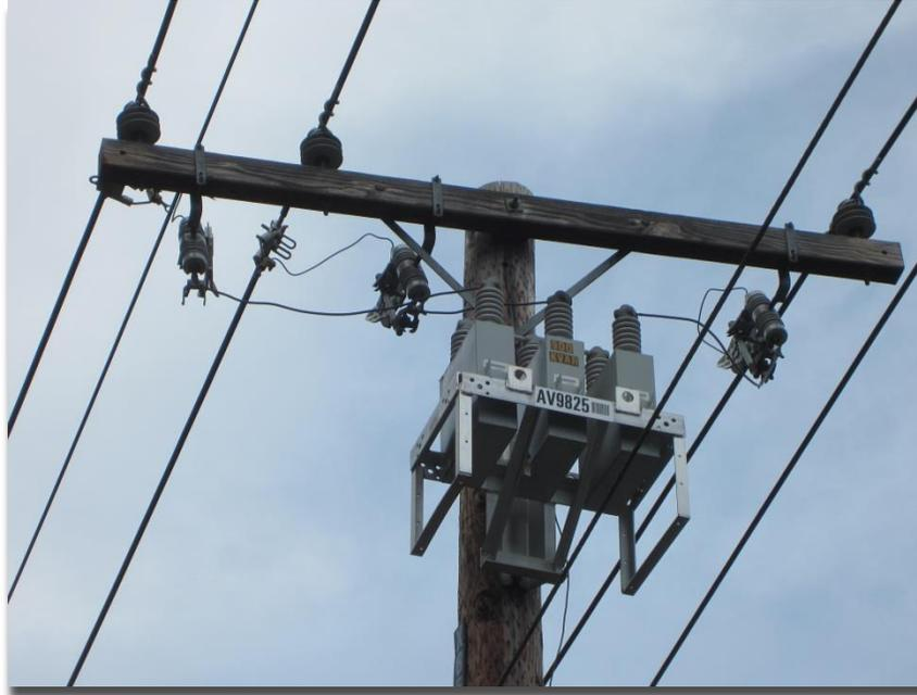
**Figure A.6. Photo of Shunt Capacitor (Photo credit: Kevin Schneider, PNNL)**
