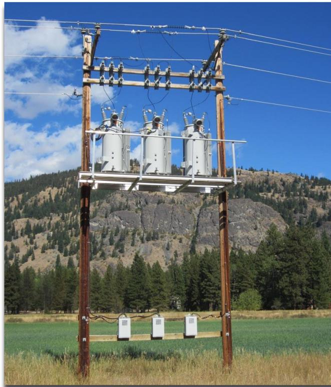
**Figure A.4. Photo of Distribution Voltage Regulator (Photo credit: Kevin Schneider, PNNL)**
