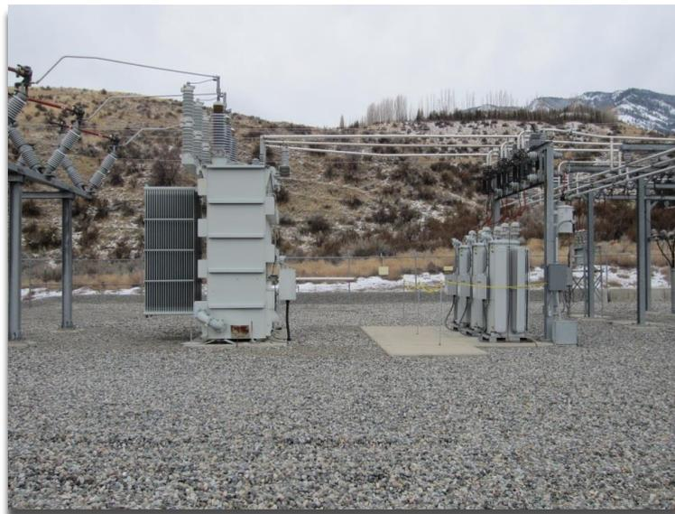
**Figure A.2. Transmission Lines Tie into a Substation Transformer (center) and Voltage Regulator (right) (Photo credit: Kevin Schneider, PNNL)**
