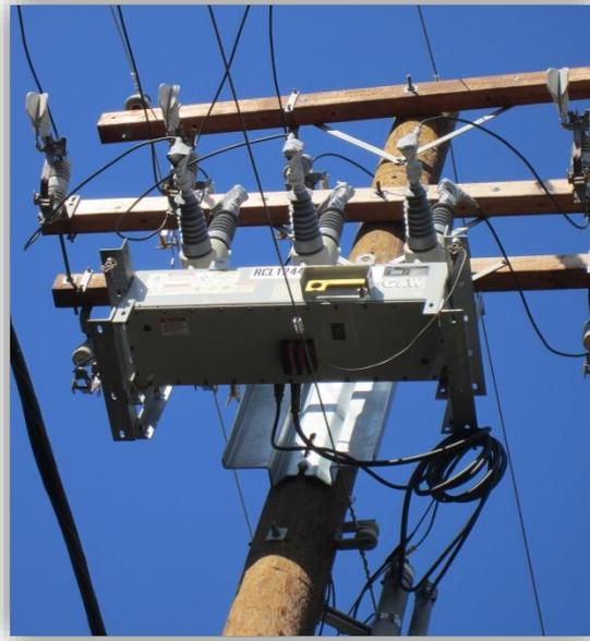
**Figure A.9. Distribution Feeder Line Recloser (Photo credit: Kevin Schneider, PNNL)**
