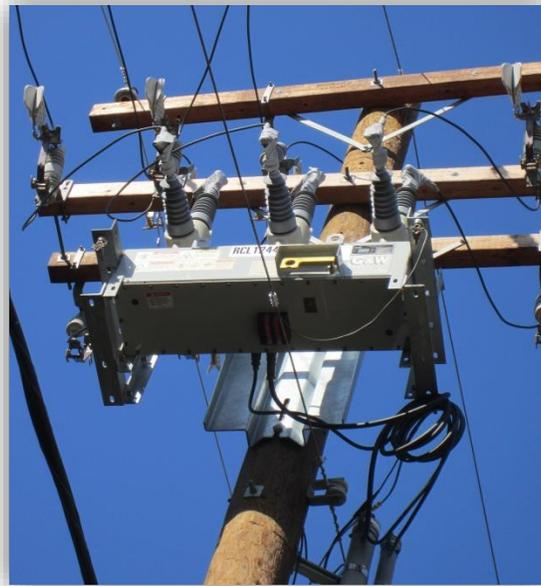
**Figure 2.13. Location of Recloser-Type Circuit Breakers on Distribution Lines**
