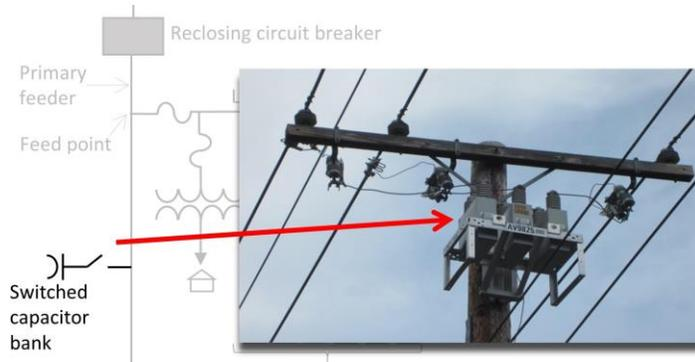
**Figure 2.15. Interconnection of a Switched Capacitor Bank to a Distribution Circuit Line**
