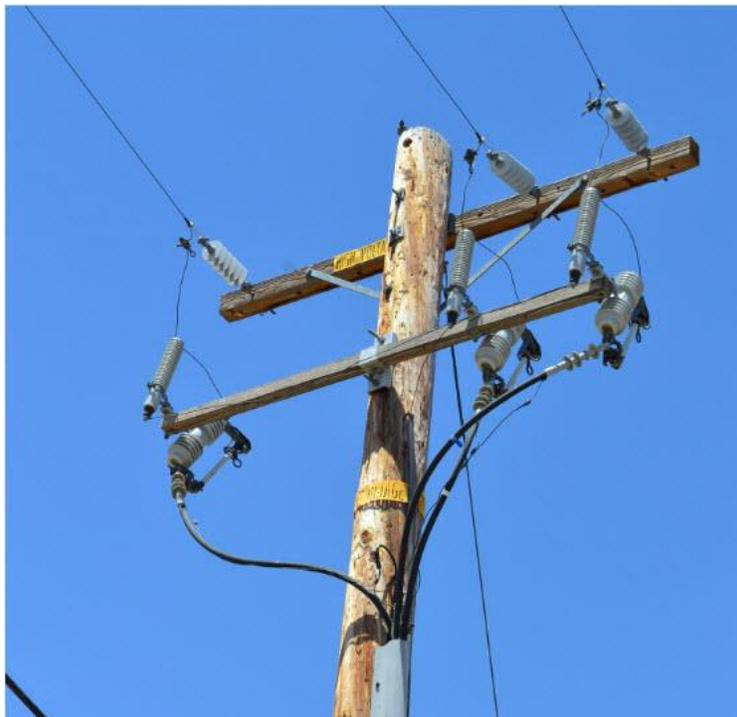
**Figure A.7. Three-Phase Line Fuses with Lightning Arrestors between Fuse and Overhead Line (Photo credit: Mike Hoffman, PNNL)**
