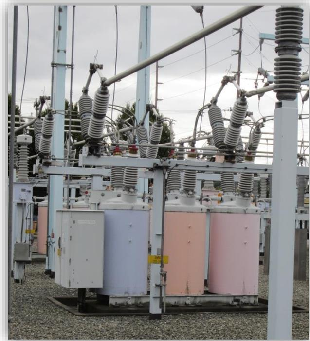
**Figure A.8. Circuit Breaker: Able to Interrupt Fault Current and Disconnect Feeder Line Faults from the System (Photo credit: Kevin Schneider, PNNL)**
