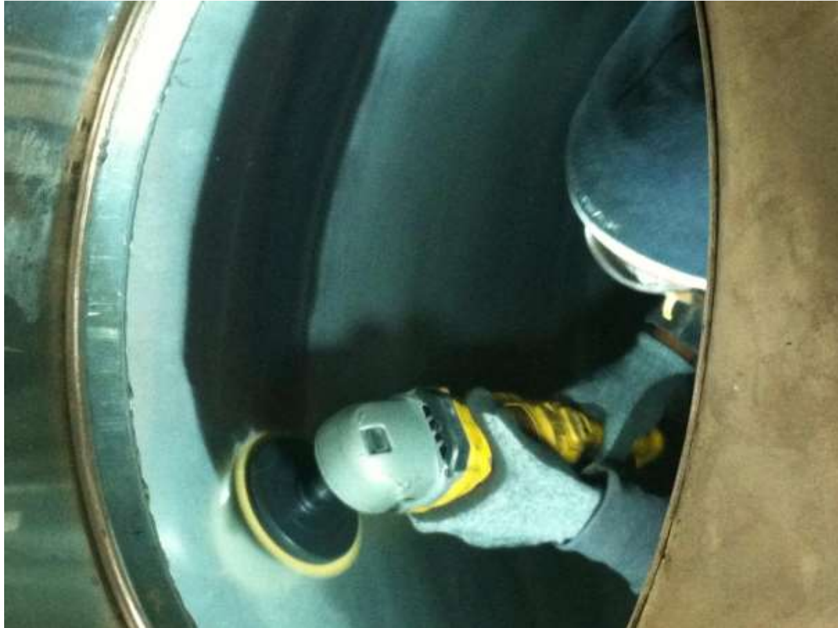
MP technique performed in-situ in vessel
