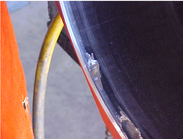
PITS PREPARED FOR ESD REPAIR
