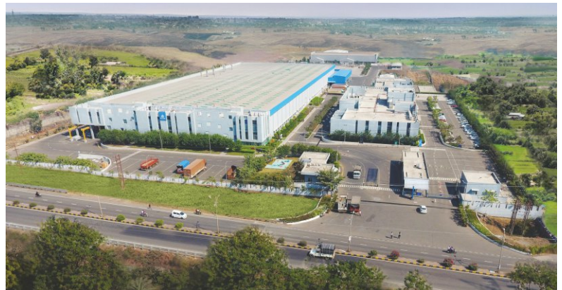
State-of-the art, Multi-Purpose Facility at Chakan, Pune
