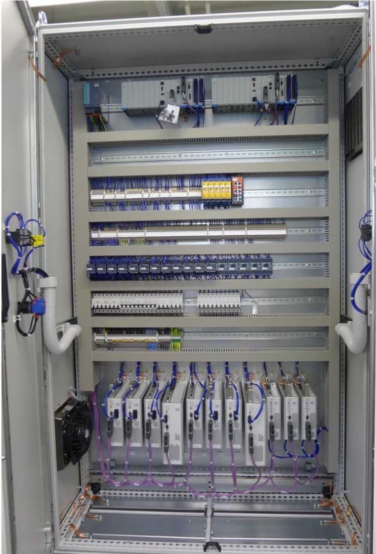
Fig. 3-20: EMC-compliant construction and installation of a cabinet with installation devices from FESTO EMC-compliant system-side wiring on cable racks and in cable trays
