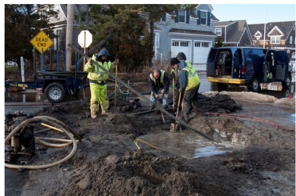
Photo: FEMA/Wendell Davis Jr.
