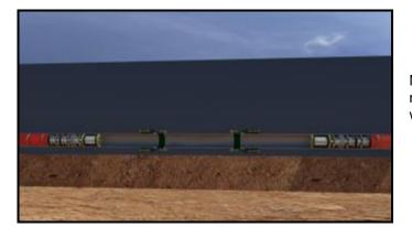
New section of pipe installed using mechanical connectors or hyperbaric weld.
