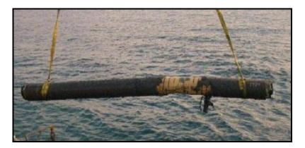
Figure 2: Cut Out Damaged Section of Pipeline
