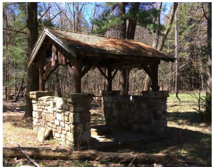
WPA Pump Shelter
