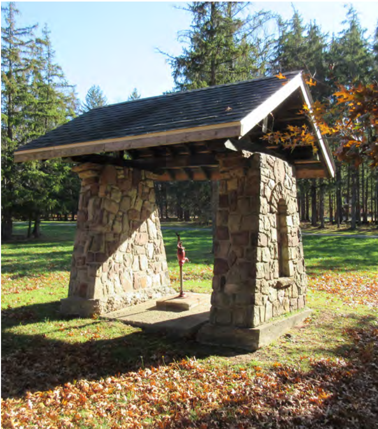
WPA era historic pump shelter
