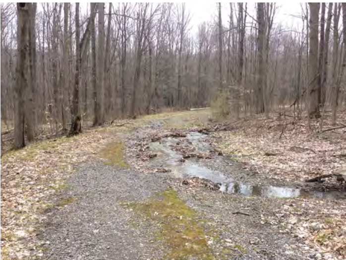
Drainage issues on the northern ravine trail
