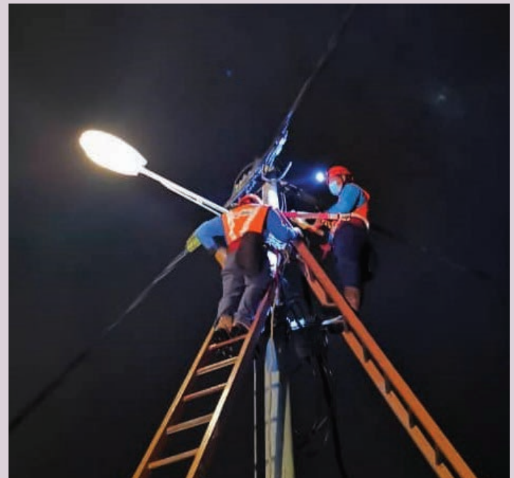
LED Streetlight Replacement Programme
